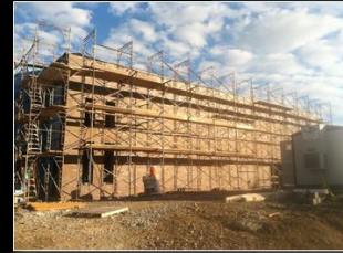
Scaffolding Congestion – Area E North Elevation
